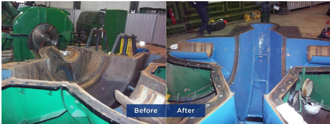
Image 1- Pump casing before and after Belzona application
