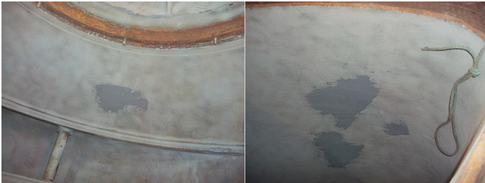
Images 9&10- Substrate rebuilt with Belzona 1111
