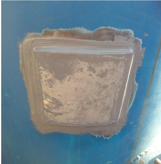
Image 3: Plate cold-bonded with Belzona 1212
