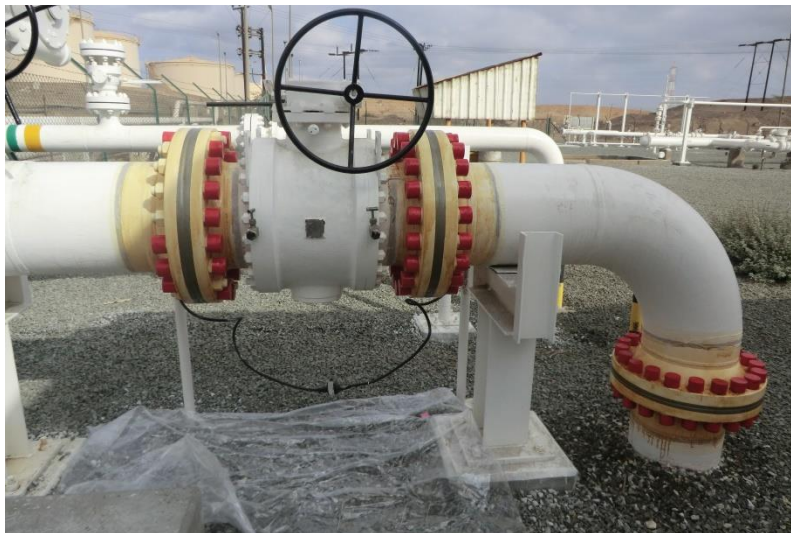
Surface prepared, Belzona 8411 applied and bolt caps installed
