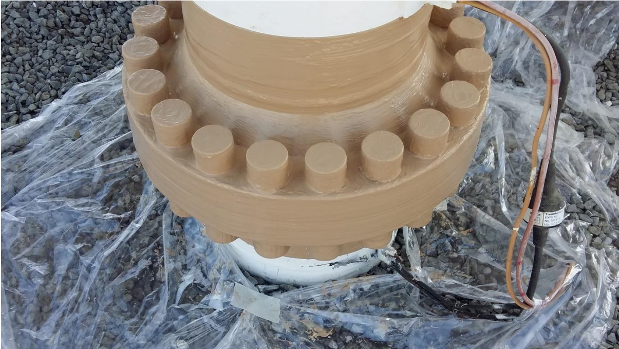
Application of first coat of Belzona 3411
