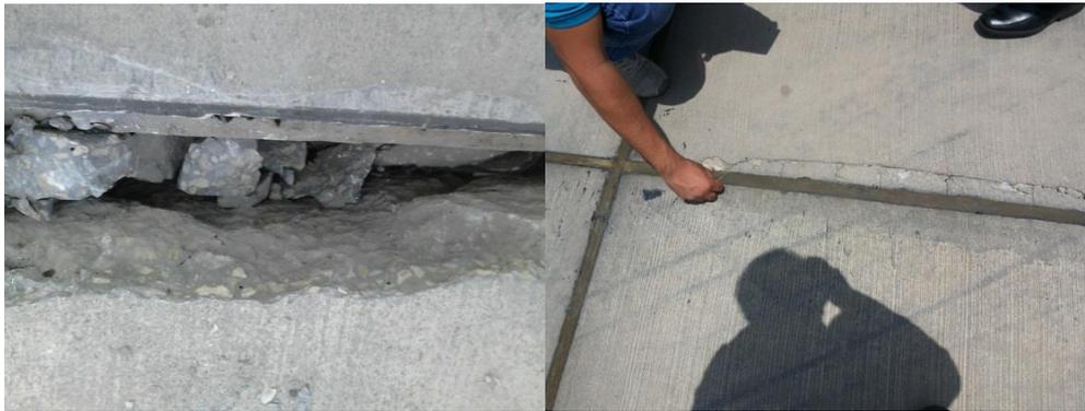
Cracked and spalled concrete
