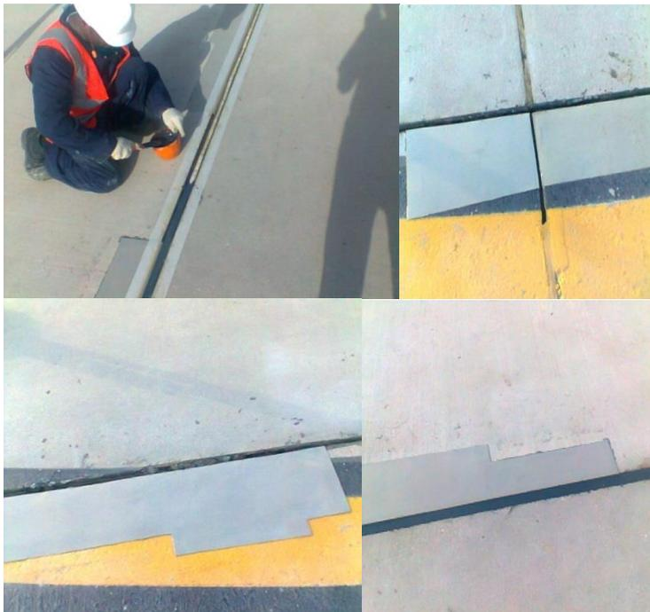
Concrete rebuilt and expansion joints installed
