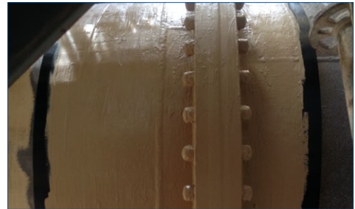
First layer of Belzona 3411 applied
