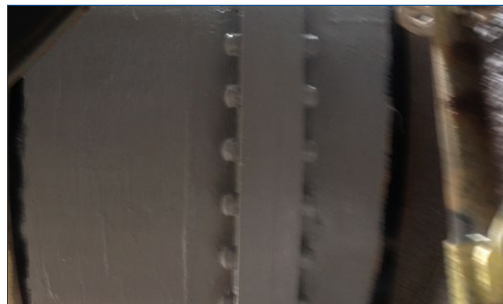
Completed application on the flange
