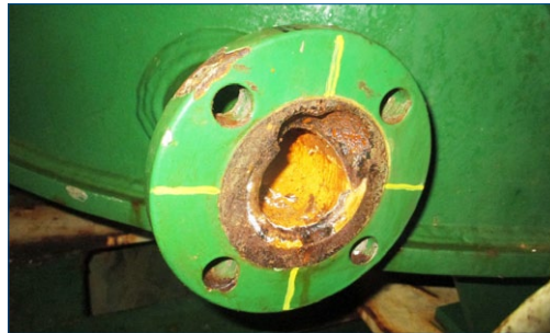
Flange face highly corroded
