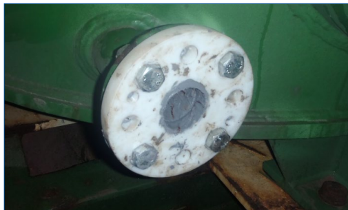
Former in place with Belzona material
