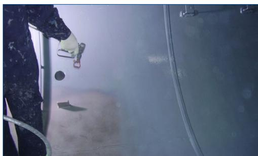
Spray applied Belzona lining
