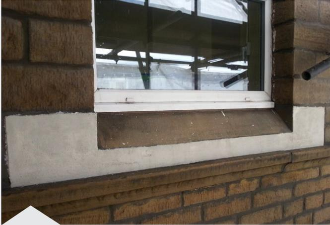
Stonework sucessfully rebuilt with hard-wearing system
