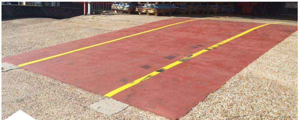
Loading bay fortified with abrasion resistant repair composite
