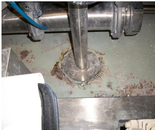
Corrosion caused by flavour oils and caustic soda
