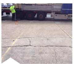
Abrasion damage on concrete substrate
