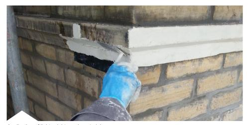
Application of lightweight repair material
