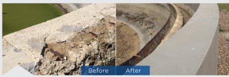
Tank wall repaired and protected with epoxy materials
