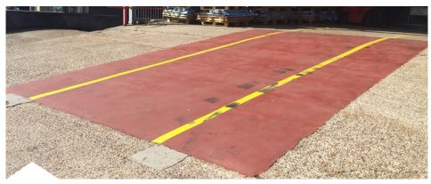
Loading bay fortified with abrasion resistant repair composite
