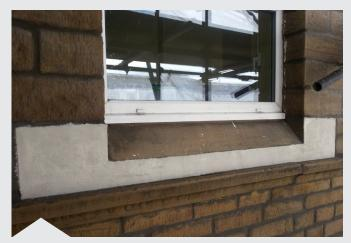
Stonework sucessfully rebuilt with hard-wearing system
