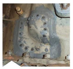
Plates bonded with epoxy repair composite
