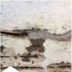
Lightweight material used to rebuild ceiling
