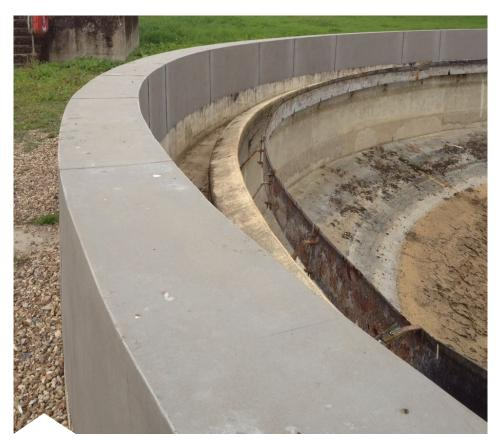
Substrate rebuilt and protected with rapid curing epoxy system
