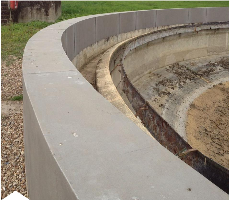
Substrate rebuilt and protected with rapid curing epoxy system
