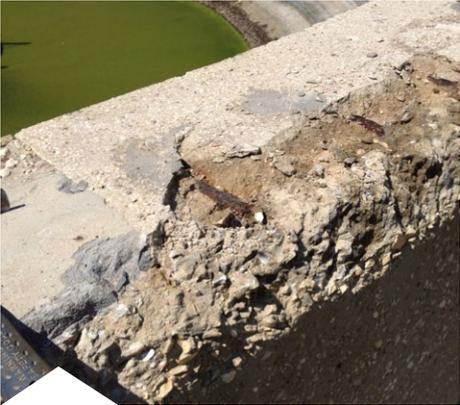
Badly eroded substrate
