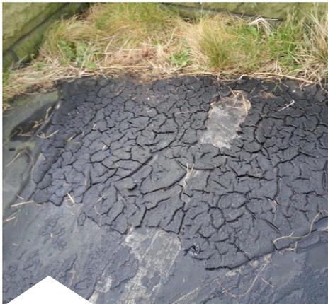
Deteriorated asphalt substrate
