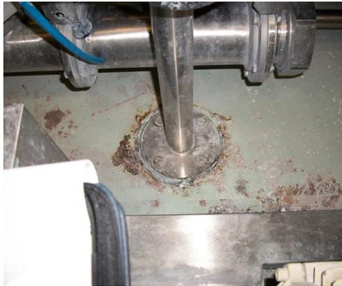
Corrosion caused by flavour oils and caustic soda
