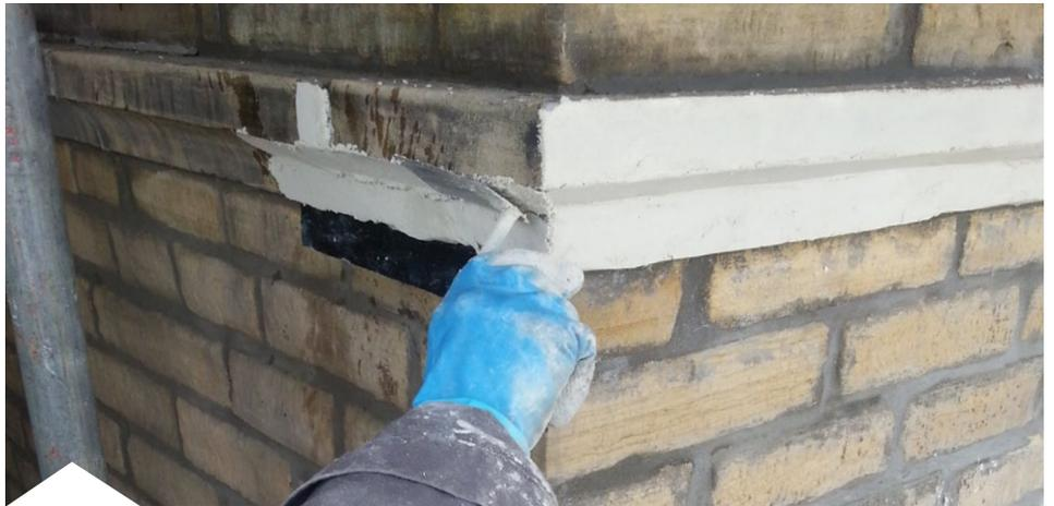
Application of lightweight repair material
