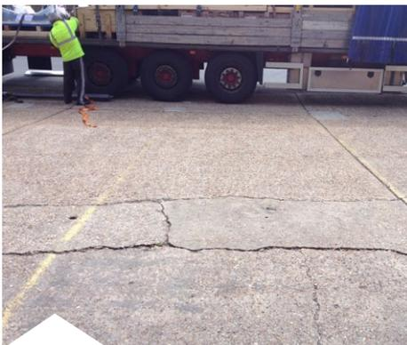
Abrasion damage on concrete substrate
