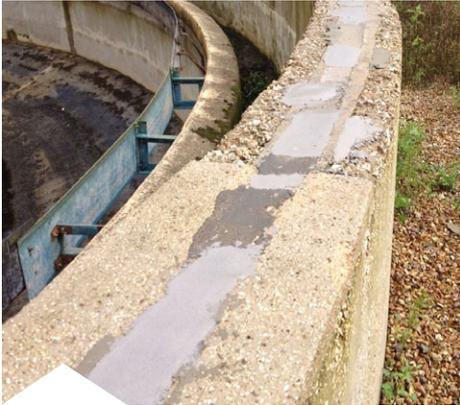
Area rebuilt with durable material
