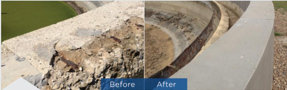
Tank wall repaired and protected with epoxy materials
