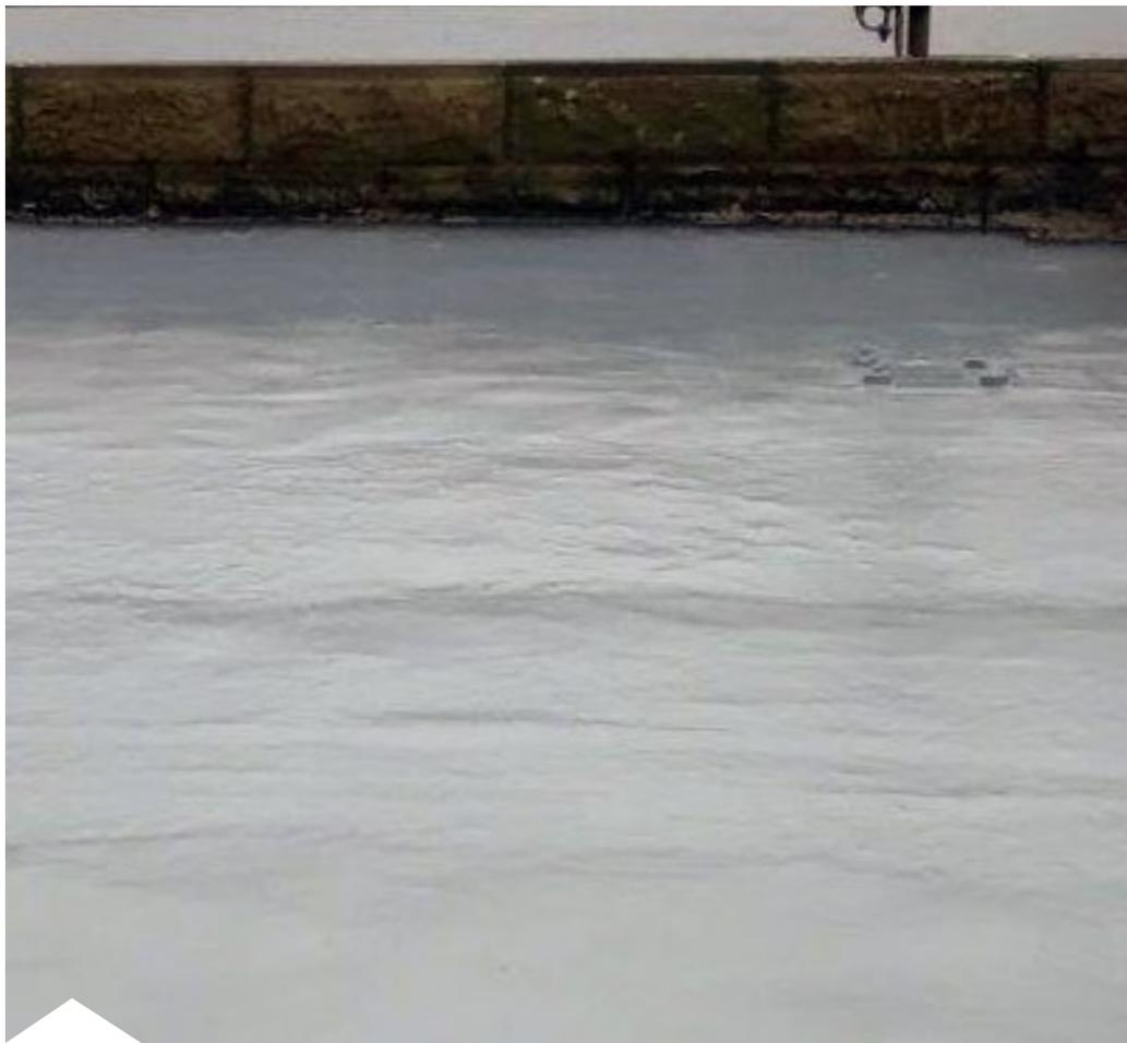
Roof repaired and protected with hard-wearing material and waterproof coating
