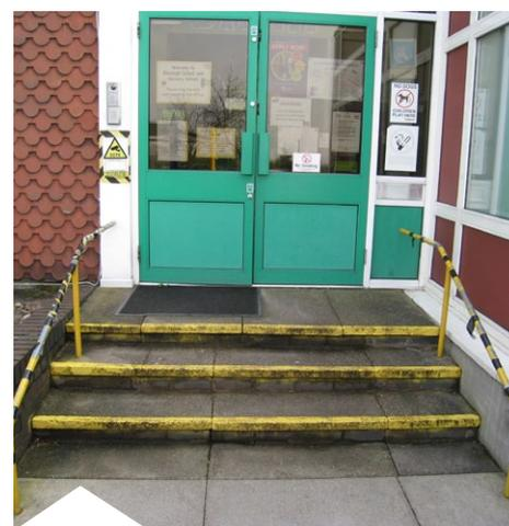
Safety grip system required for damaged steps
