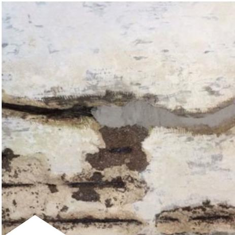
Lightweight material used to rebuild ceiling
