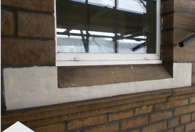
Stonework sucessfully rebuilt with hard-wearing system
