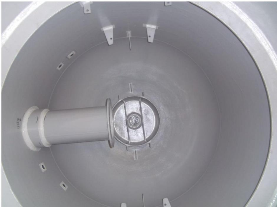
Figure 6: Belzona 1331 spray applied to a process tower in the UK North Sea for a major Oil and Gas client. The high build capacity meant that internal furniture and welds are coated resulting in minimal remedial work and faster job completion.
