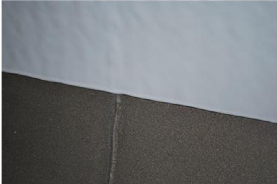
Figure 4: Single coat application of Belzona 1331 achieves full coverage of a 1.5mm high weld bead. The masking tape was removed to reveal the weld bead.
