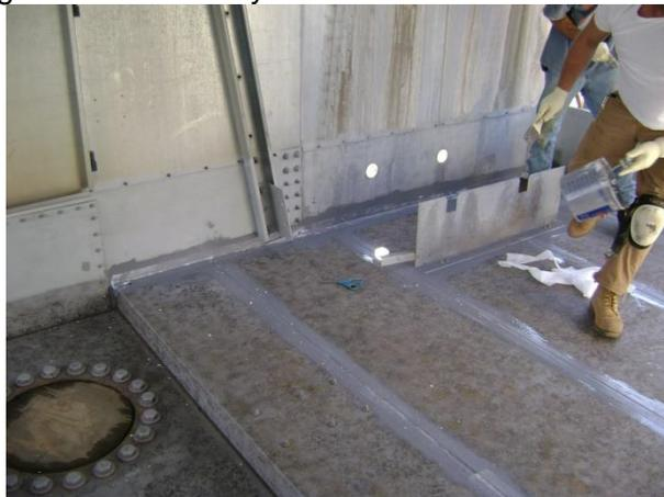
*Repair of leaking seams using Belzona waterproofing membrane*
