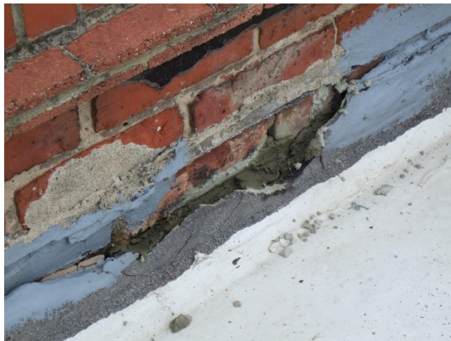
Roof flashings can prove problematic due to the amount of dissimilar materials
