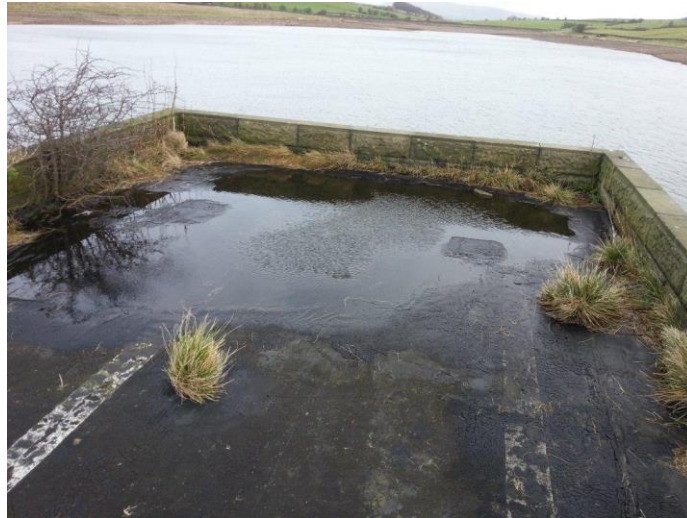
Flat roofs are prone to pooling
