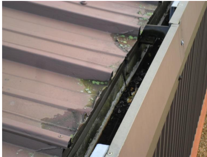
Metals seams are often neglected and can develop cut-edge corrosion
