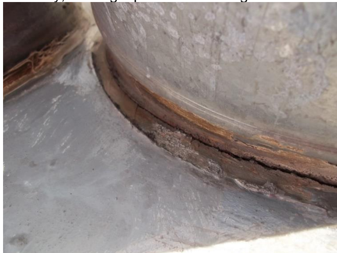
Over time, rubber roofing materials can become brittle and crack
