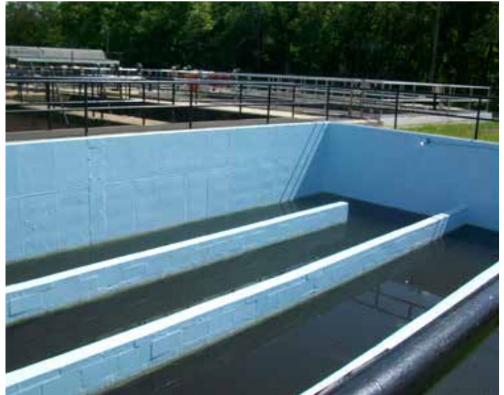
Belzona 5111 used for wall protection of a chlorine tank
