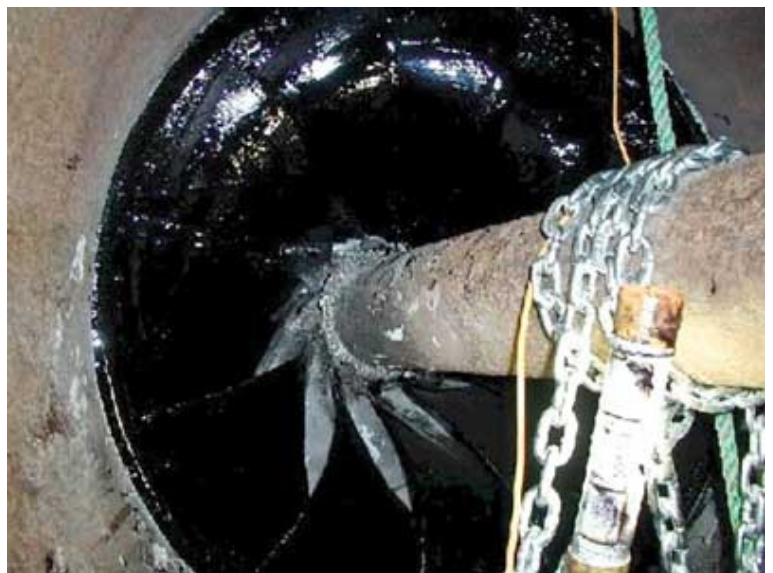
Figure 9 - Well-dressed impeller. A cavitation-resistant elastomer coating was applied to this pump impeller after the impeller was returned to OEM specifications. Courtesy: Belzona Inc.
