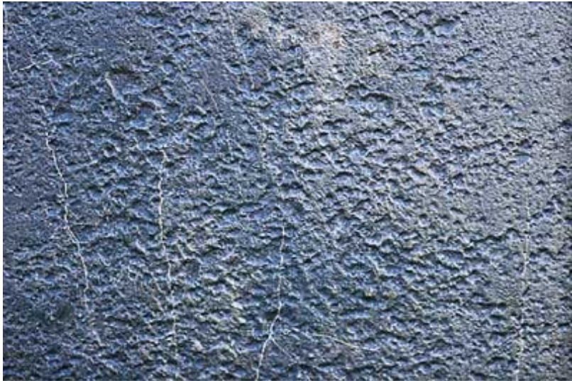
Figure 8 - Cavitation damage is severe. Close-up of damage to a pump impeller caused by cavitation. Courtesy: Belzona Inc.
