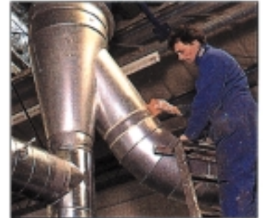
SEAL SPLIT DUCTING
