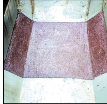
Application completed with the Belzona® 1811
