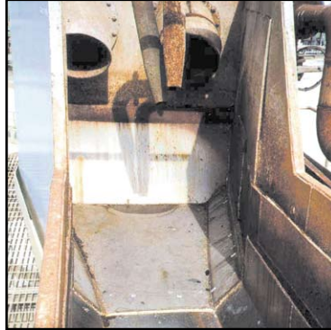
Equipment prior to surface preparation
