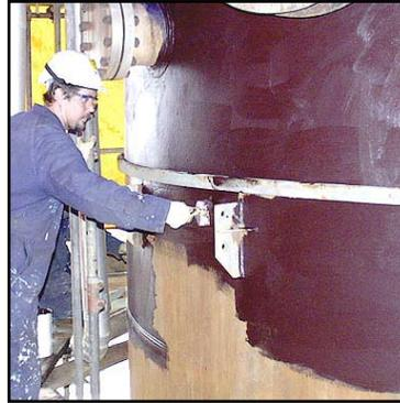
*Belzona® 5851 is easily applied to hot surfaces by trowel, brush, or even spray.*
