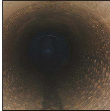
Degree of corrosion evident on the delivery tubes
