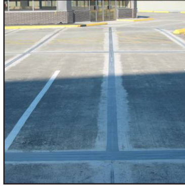
Application of 2nd coat in progress
