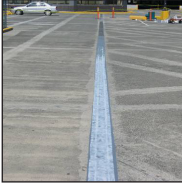
Application in progress - 1st coat with Reinforcement Sheet in place
