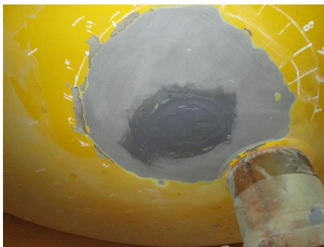
Caption: Belzona SuperWrap II applied as per engineered design
