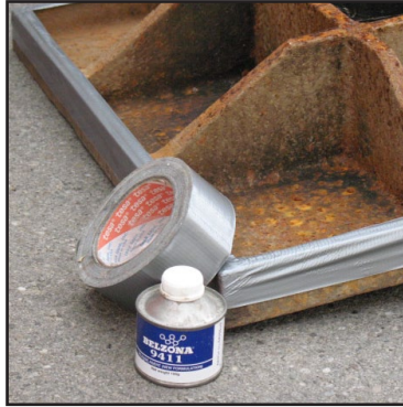
Applying Duct tape and Belzona® 9411
