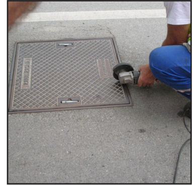
Manhole in place and position marked
