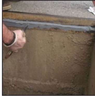
Rebuilding manhole cover seat with Belzona® 1111
