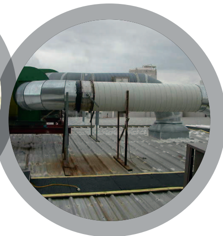
Exhaust Ducting
